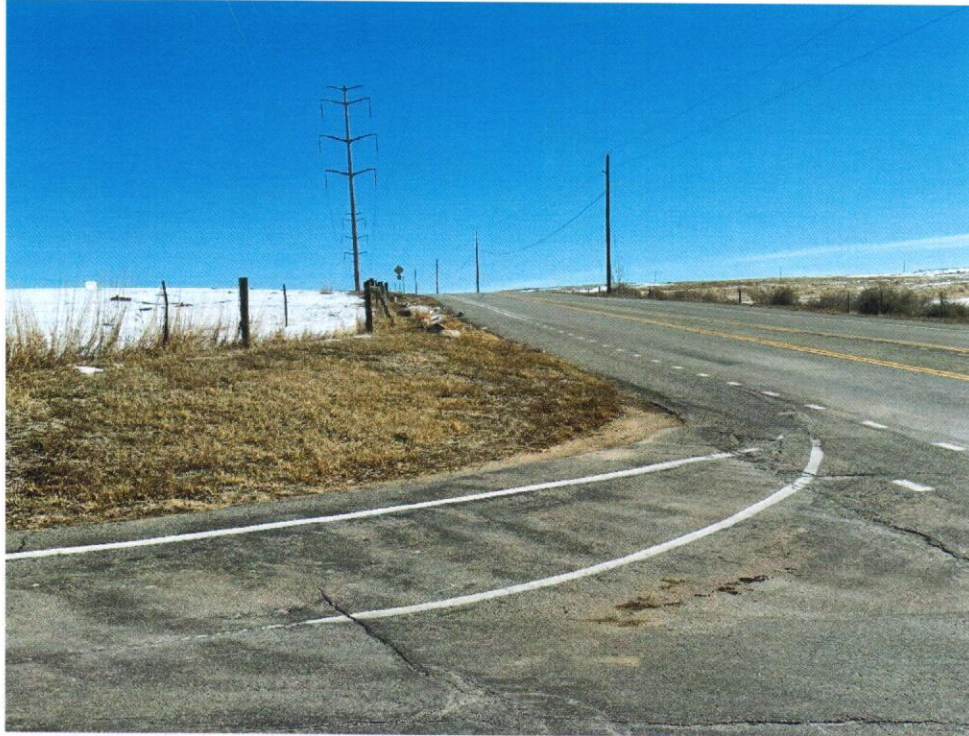
Photo 7: Poor sight distance for southbound vehicles on 79 th Street when turning out onto Lookout Road. Cars coming westbound over this hill are traveling at 50 mph or more. Does not meet recommended minimum intersection sight distance in AASHTO design guide.
