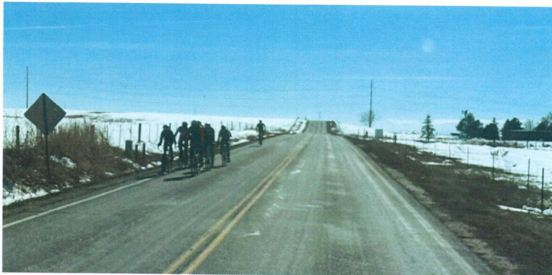
Photo 10: N. 79 th Street is regularly used for training rides, even with the multiple locations of poor sight distance due to vertical curvature. Unfamiliar motorists accessing the tennis center may not appreciate the danger of passing bicyclists with the limited sight distance of oncoming traffic.
